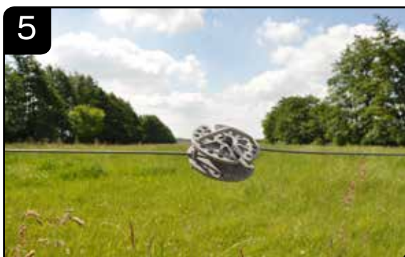
5 Fit and tension the fencing
