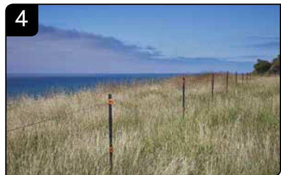
4 Fit the intermediate posts
