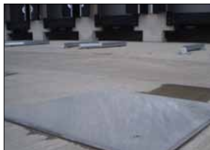
TP 20 - SURFACEFIX 1000mm x 1000mm Surface mounted with a bevelled edge.
