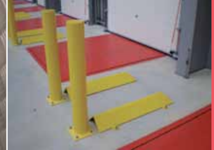
DOCK RAIL GUIDES
