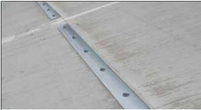
WS-30 150 x 150 angle iron wheel stop 3 metres long.
